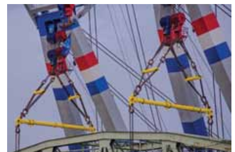
Fig.15 Combination of Spreader and lift beams
